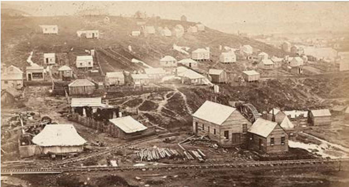
The view from Irishtown overlooking Block 27 to the right.
