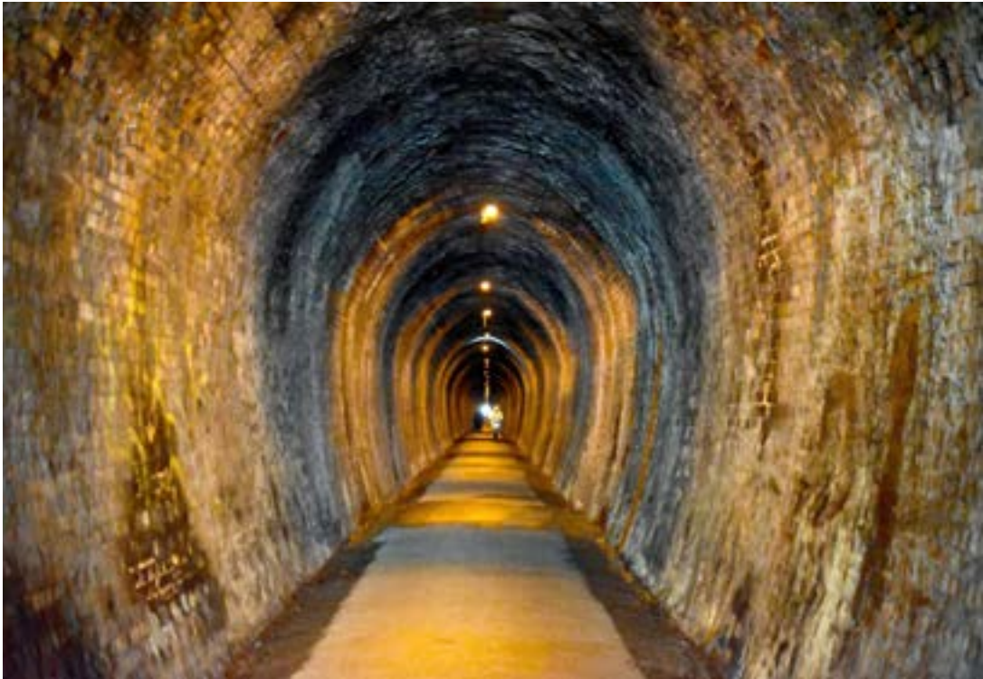
Repairing the Karangahake Tunnel is the trust’s immediate priority.
