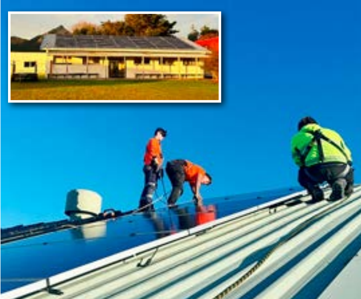
Solar panels are installed at Harataunga Marae, Kennedy Bay. Photo: SUPPLIED
