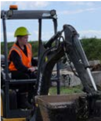
Lexis operates the digger.
