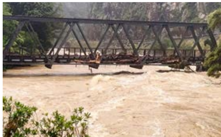
Up to $4.38 million will be spent on repairs to the Ohinemuri River Trail.
