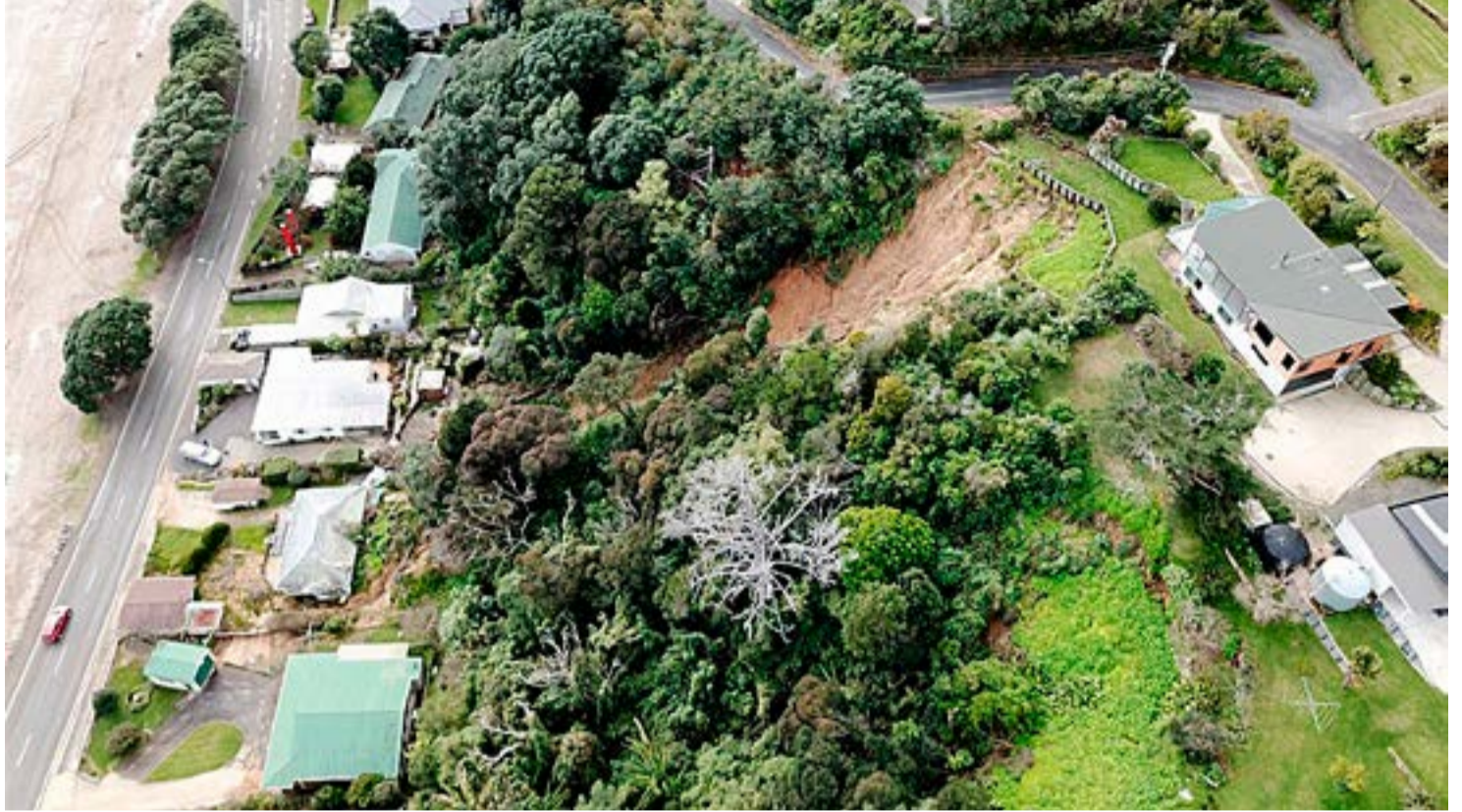
The early-2023 storm caused a large slip on to multiple private properties at Thornton Bay on the Thames Coast.
