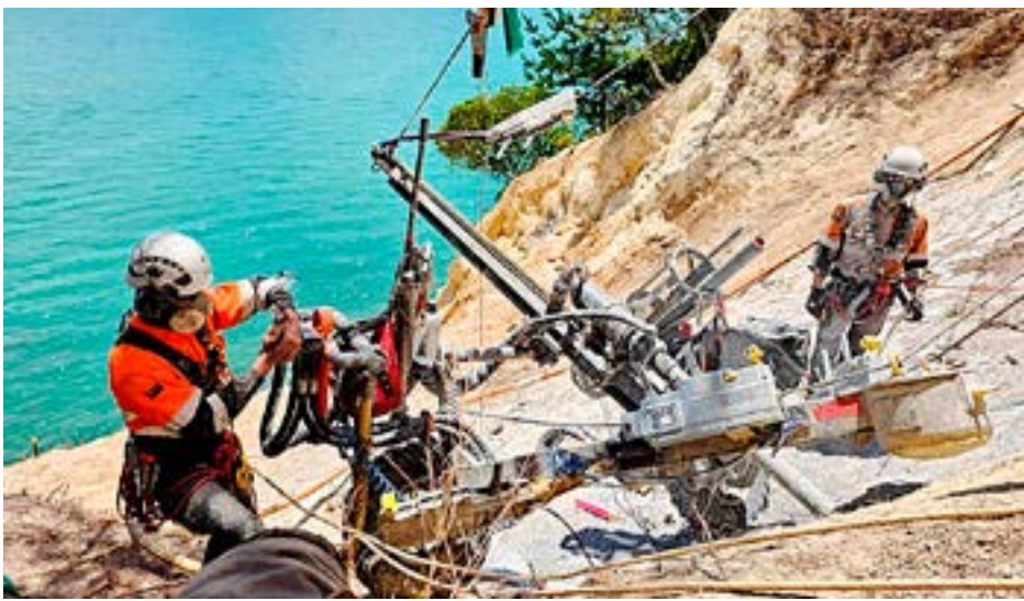
Recovery works include intermittent road closures at Ruamahunga Bay. Photo: SUPPLIED
