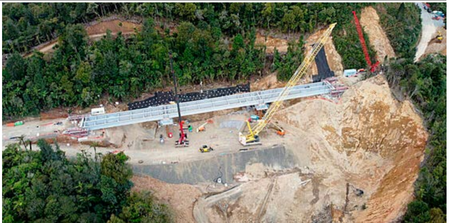
The final beam (girder) was lifted into place on October 18.
