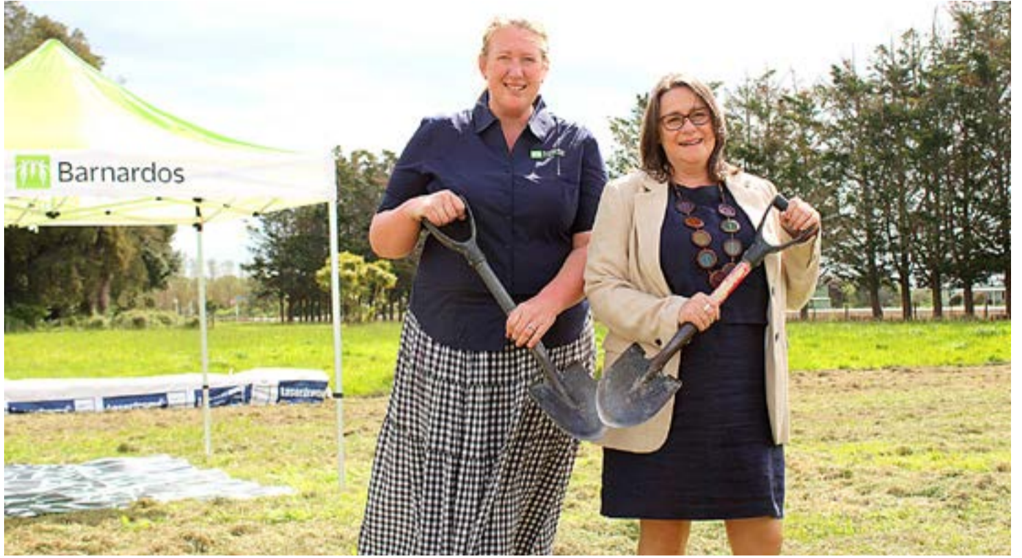
Beccs Aislabie and Heather Taylor stand at the new Barnardos site with shovels ready.
