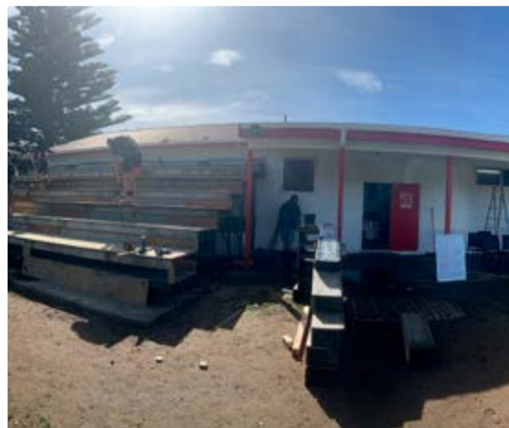
Work is underway at Whangamatā Rugby Club.
