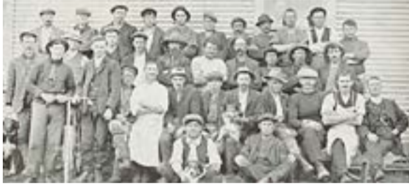
Some of the men carrying out the electrical scheme at Horahora.
