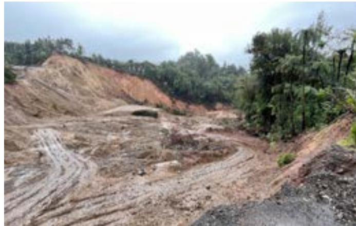
Budget 2023 includes funding aimed at cyclone recovery, and building future infrastructure resilience. Photo: SUPPLIED/WAKA KOTAHI
