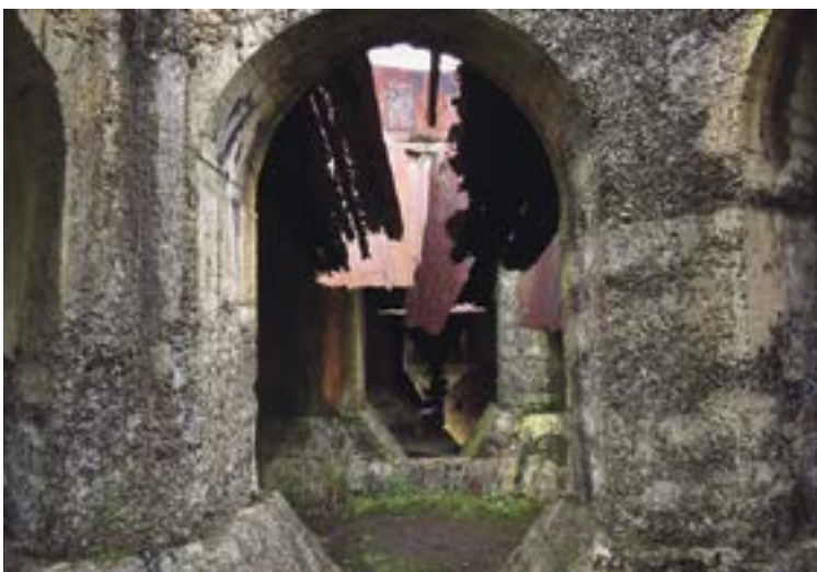
The foundations of the cyanide tanks still remain at the battery; an exciting place to explore or play hide-and-seek.
