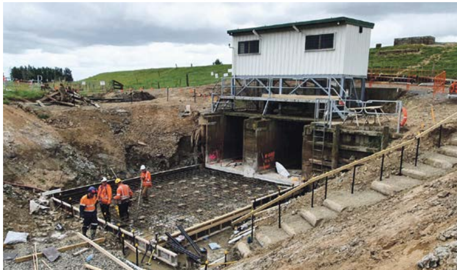
The pump station at Mill Rd, Paeroa, is part of Waikato Regional Council's flood protection infrastructure that falls under the draft sustainable infrastructure decision making framework. The Mill Rd pump station was recently upgraded together with the Roger Harris pump station, which are both critical in providing flood protection of the Paeroa community. The project cost $4.5 million, including $2.88m from the Ministry of Business, Innovation and Employment, and created 13 jobs over 20 months. The pump stations allow for primary use of land that's lower than the mean high tide level, and remove rain and flood waters to an agreed height. The work includes upgrading inlet bays, screens, handrails and platform access. The four pumps at the Mill Rd station combined give the largest protection in New Zealand, pumping 10.4m 3 per second. The Roger Harris pump station pumps 4.4m 3 per second.
