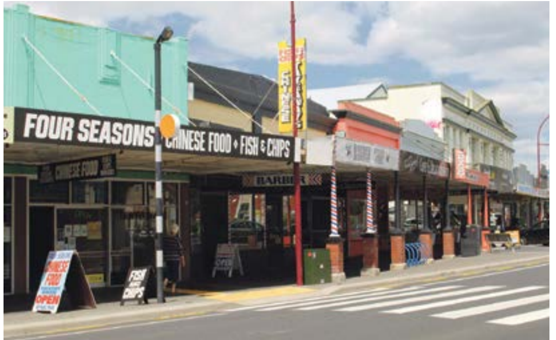
Unreinforced masonry buildings on Paeroa's central business district have been deemed an earthquake risk.
