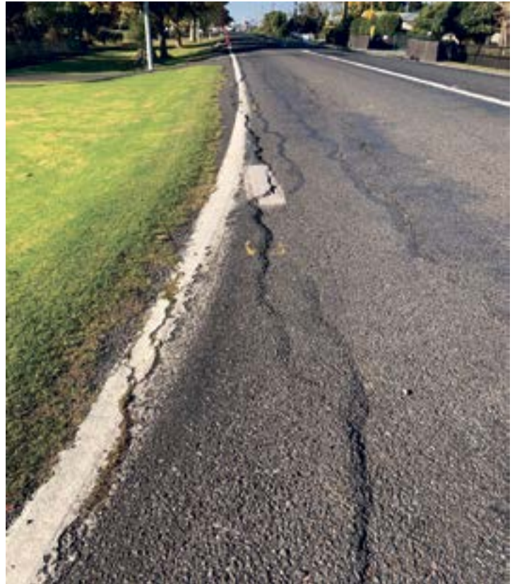
Council expects work to repair Pipiroa Rd will begin after October.
