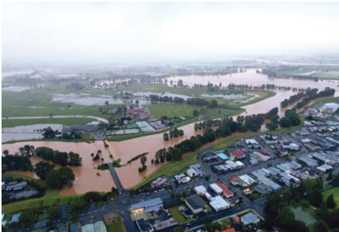
The network of stopbanks surrounding the Hauraki district protected Paeroa from flooding during the severe weather events of 2023.
