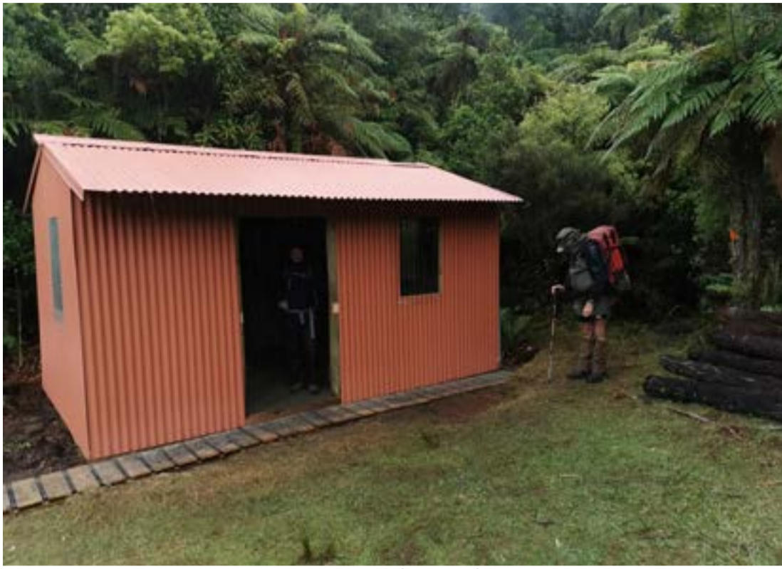
The Wairoa shelter now has coloursteel walls and roof, a gravel floor, polycarbonate windows and a seat constructed from leftover timber.
