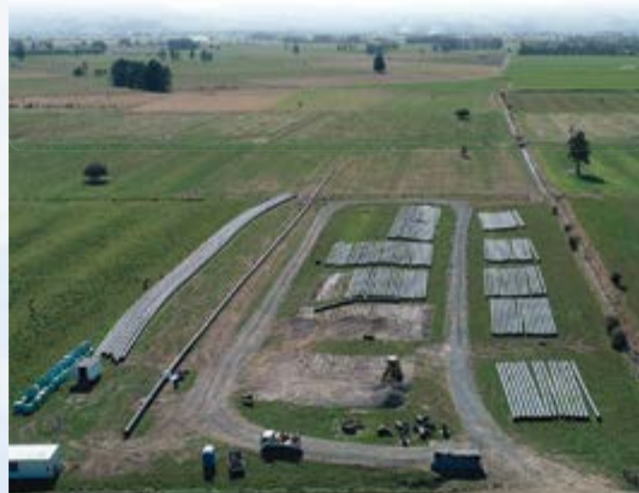
Kerepēhi raw water pipeline renewal
