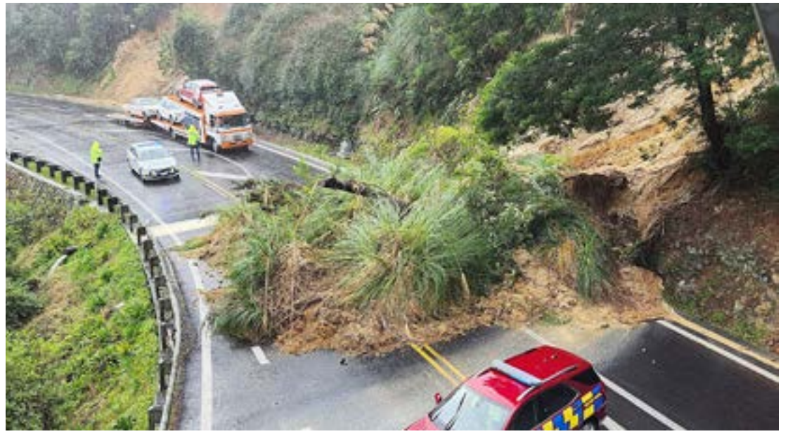
The slip in Karangahake Gorge closed the road for several hours last week.
