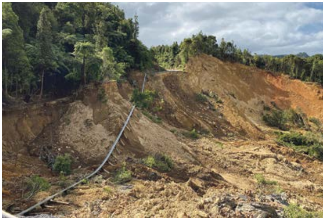
The slip on SH25A now measures around 110 metres across and is highly unstable, Waka Kotahi says.
