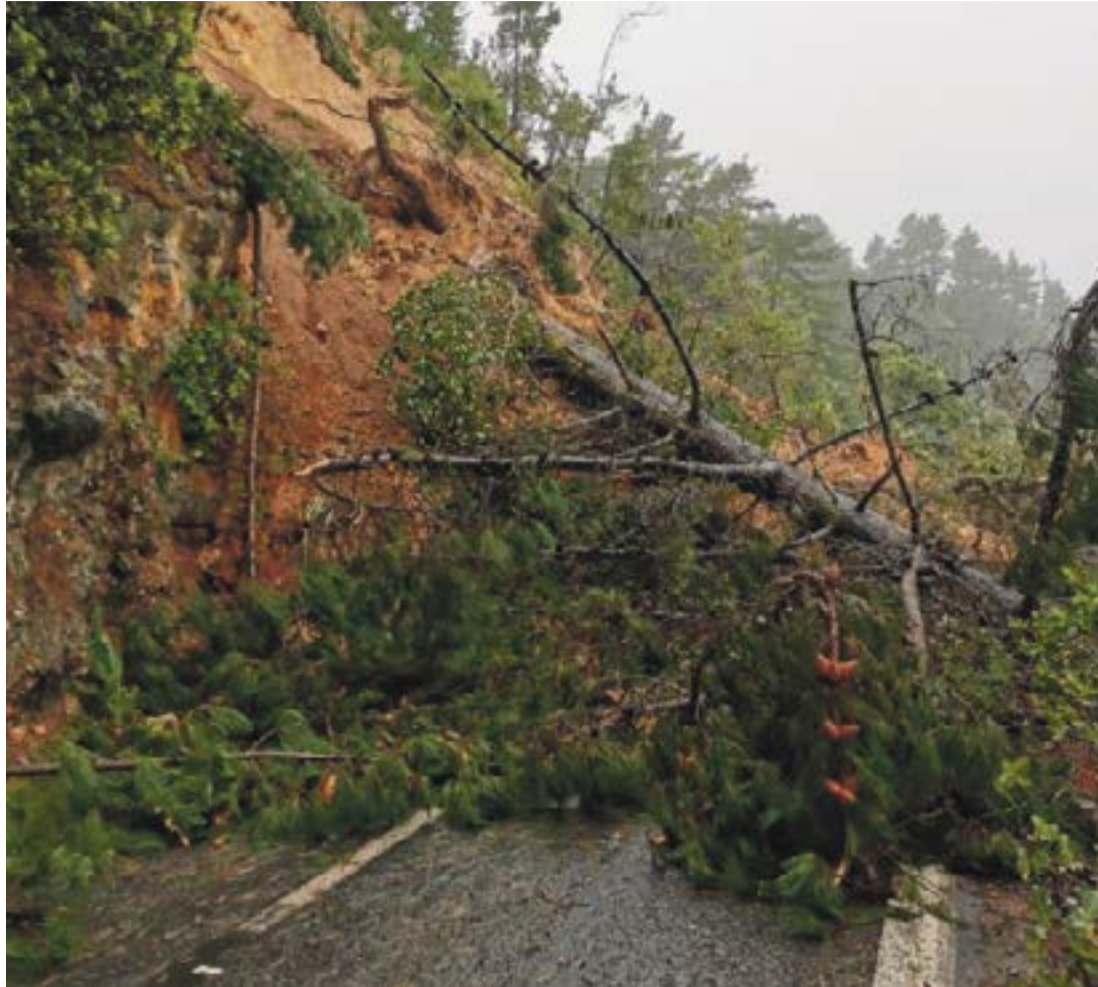
The Thames Coast Rd was among several Coromandel roads that were closed last week after slips.
